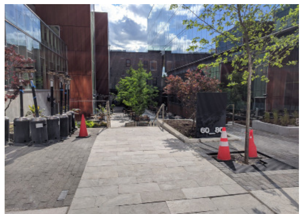
Photo 6: Nestled between 60 and 80 Atlantic Avenue, a contemporary take on the distinctive courtyard spaces
