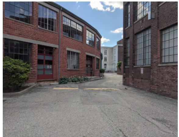
Photo 5: Example of a characteristic Liberty Village mid-block passage way
