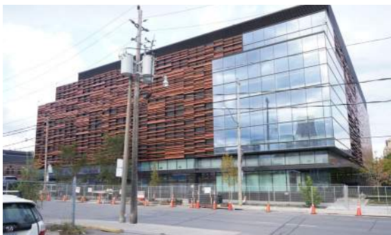
Photo 29: Equinix Data Center (8)
