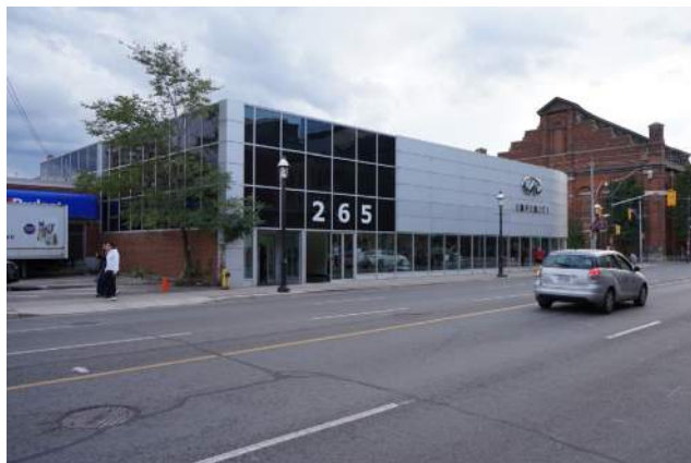
Photo 23: Front St. East & Berkeley St, looking southwest
