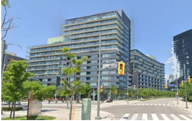
Photo 10: Bayview Ave., looking north
