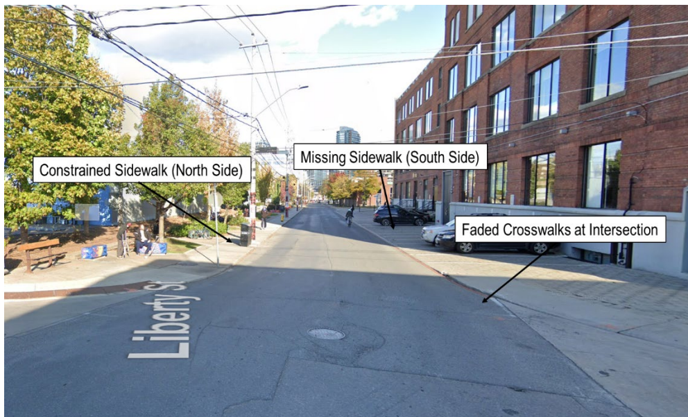
Figure 2-4: Liberty Street / Fraser Avenue Pedestrian Facilities (Facing East)
