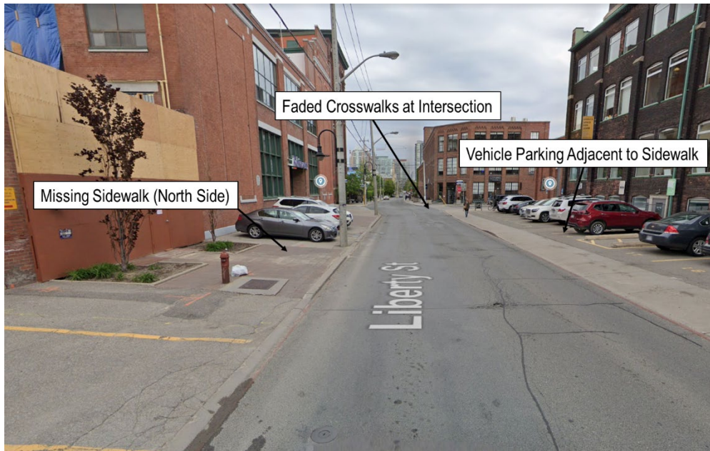
Figure 2-5: Liberty Street Pedestrian Facilities (Facing East Towards Mowat Avenue)
