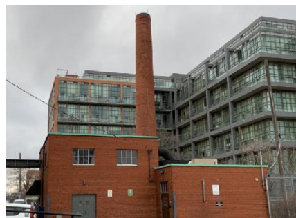
Heritage industrial elements on site (Atlantic Site)
