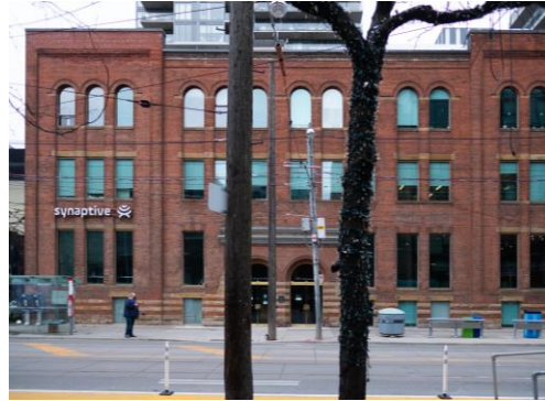
668 King Street West (Listed)
