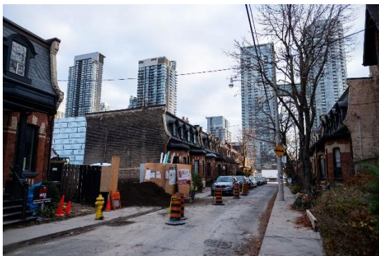
Duncan Street, looking south
