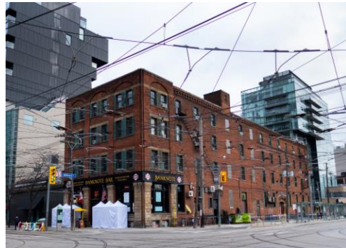
663 to 665 King Street West and 69 to 73 Bathurst Street (Designated)
