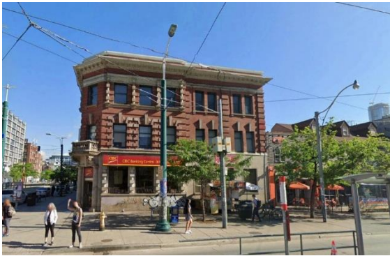
370-372A Queen Street West
