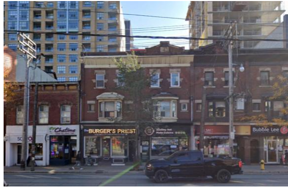
459-469 Queen Street West
