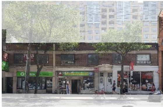
449-453 Queen Street West
